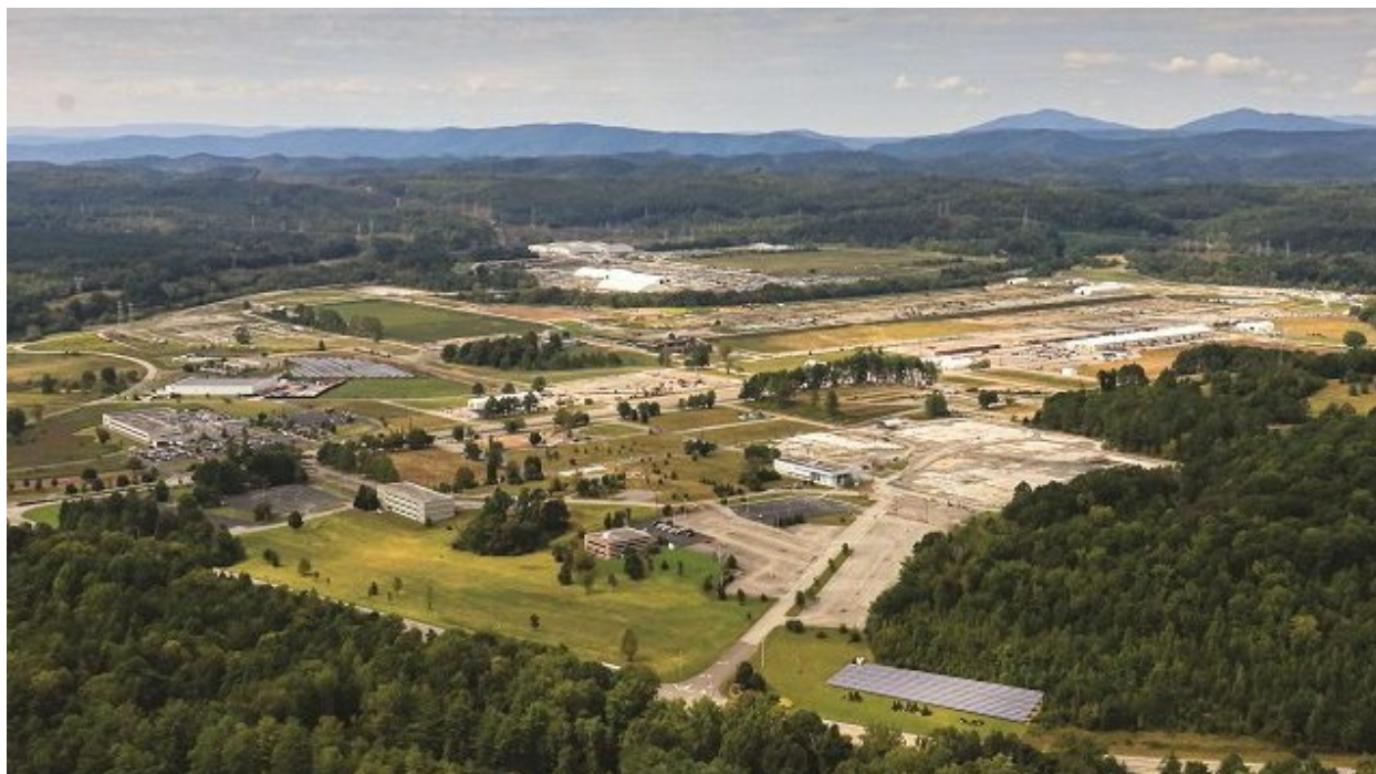
Figure 1.9. Aerial view of East Tennessee Technology Park
