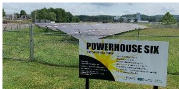
Figure 3.4. Oak Ridge Powerhouse Six Solar Farm
